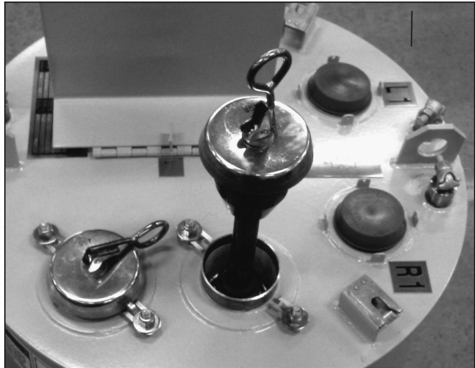
▲ Canister fuses incorporate a provision for hookstick removal and replacement.
