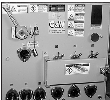
▲ Switch with front mounted fusing.
