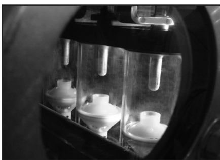
▲ Three phase visible position of contacts.
